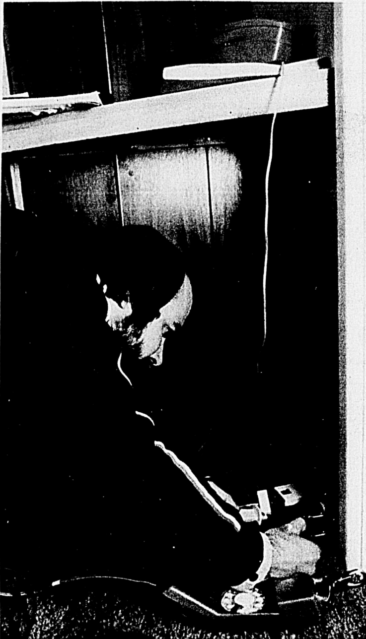
Repairman Williams checks out a telephone jack.
