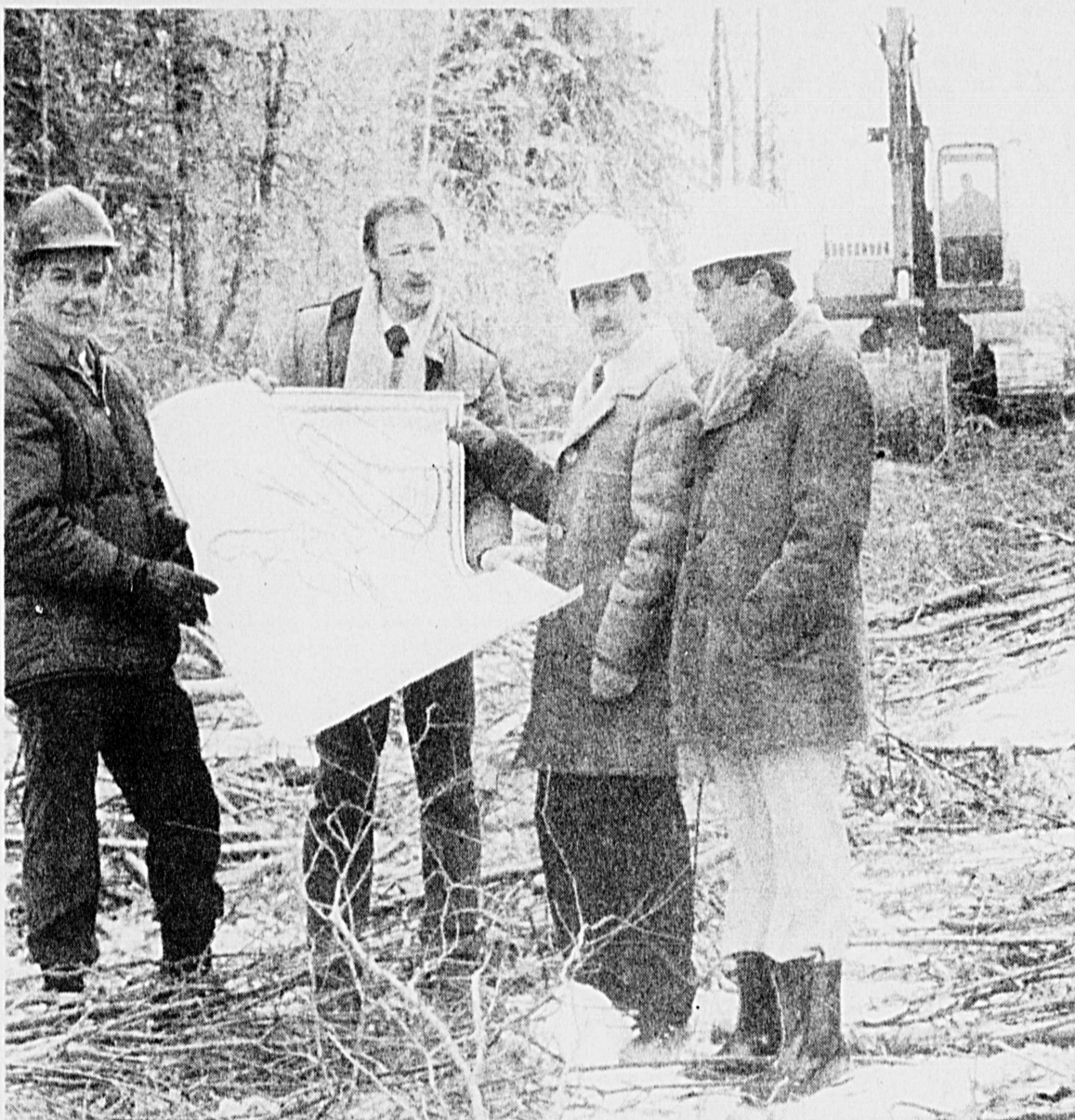
Marking the start of construction for the Trees for the World project, Steve Marynovich from the Prince George East forest district, committee
