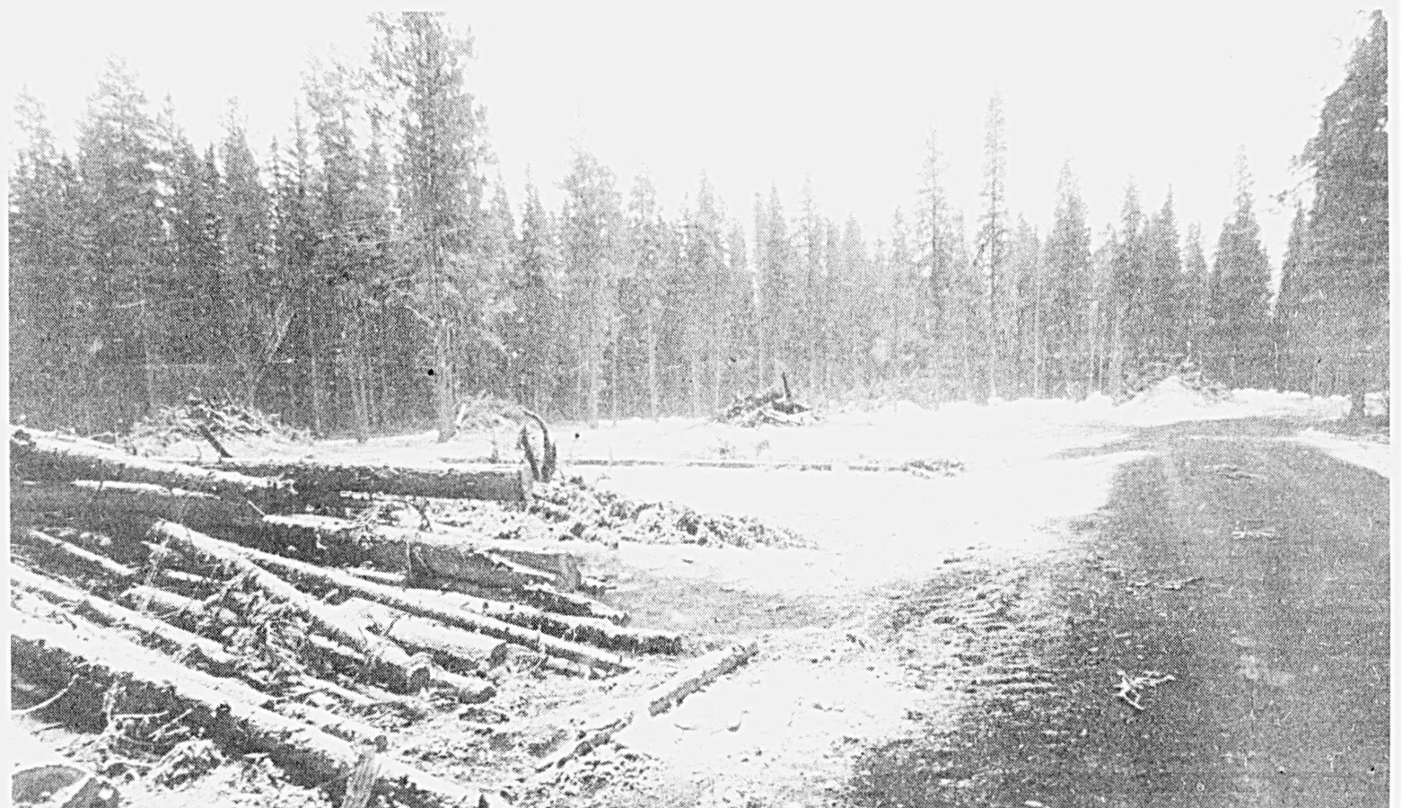
Development of large lots in Sykes Subdivision continues.
